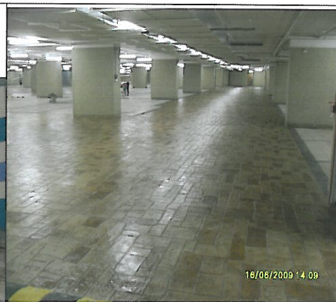
Carpark Polymer Stamp Concrete Flooring 停車場地台印花
